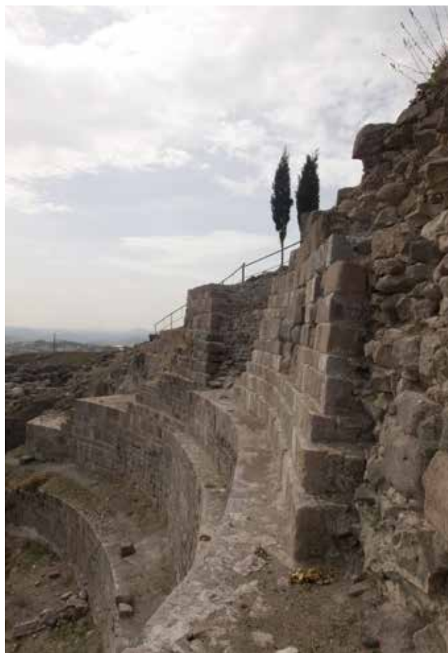
ABOVE: Odeion retaining walls after restoration work OPPOSITE: Terrace retaining wall: before and after restoration work
