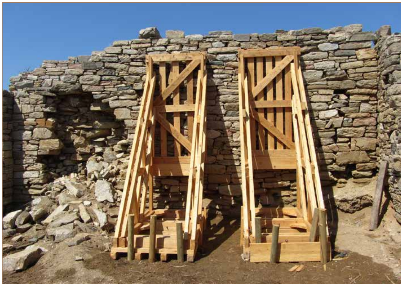
ABOVE: Timber reinforcements in the Magasin des colonnes OPPOSITE: Courtyard of the Magasin des colonnes, before and after cleaning
